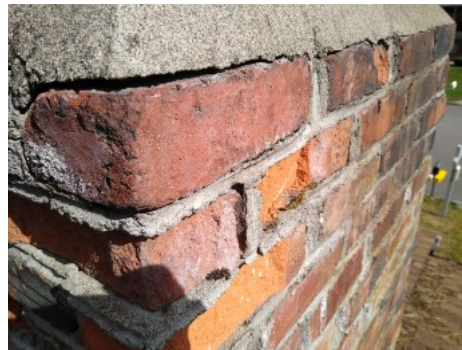
deterioration of brick and mortar
