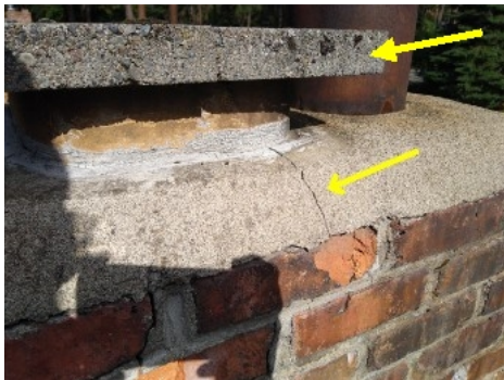
minor cracking and blocked flue
