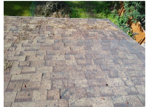
slight granule loss on this portion of the roof
