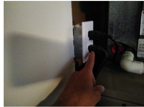
electric shut-off
