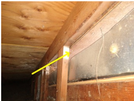
missing siding and sheathing
