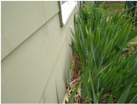
vegetation in contact with siding
