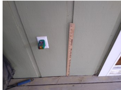
open ground condition
