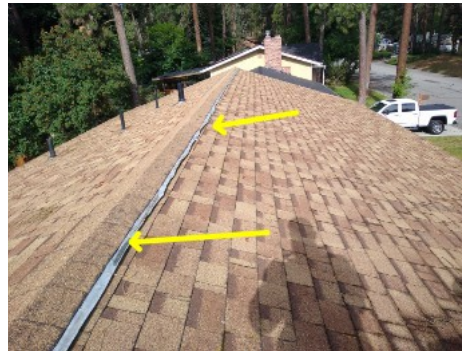
zinc strip on the ridge will help prevent some moss growth but will not guarantee no moss growth
